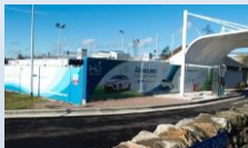
Second HRS Opening of ACHES - increased the hydrogen supply and offered hydrogen resilience for the City
